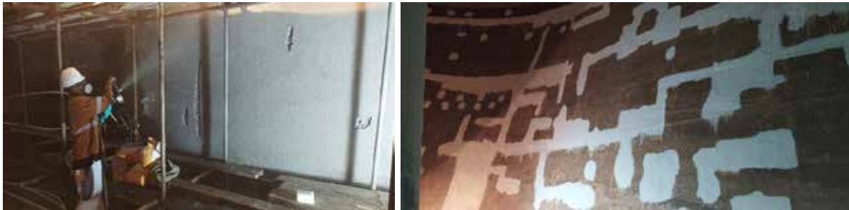
Figure 7: Final coating of Sikagard PW in Unit 3 spiral case
