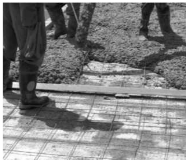
Pumping a concrete topping onto precast flooring. Reinforcement and screed battens in foreground.
