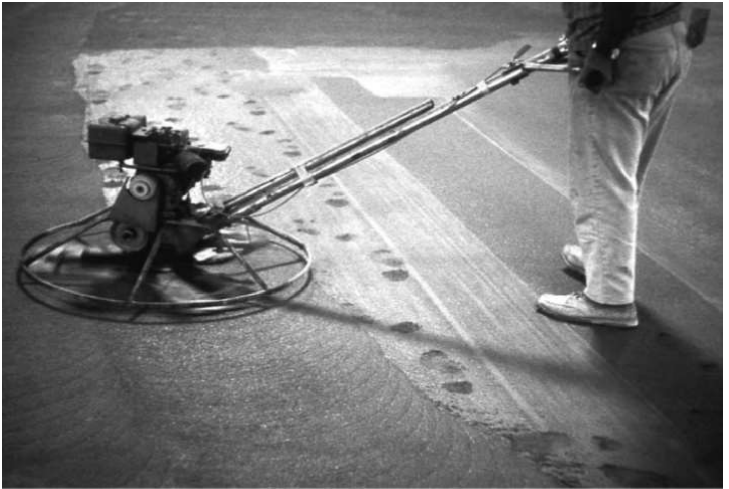
Power floating a screed.
