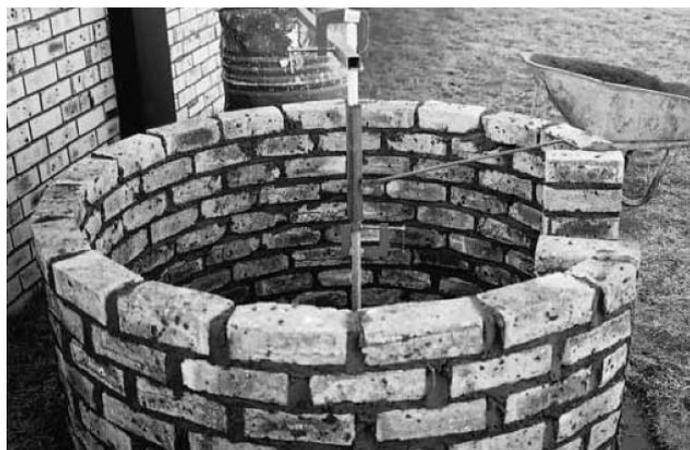
Although this takes time to set up, it makes accurate brick laying much quicker. (See photograph above right.) Unless the base will be plastered, a pointing tool is now used to finish the mortar between the bricks. To improve bond between bricks and mortar and make brick laying easier, clay bricks should be pre-soaked. If 'cement bricks' are used for the base, they should be laid dry.
